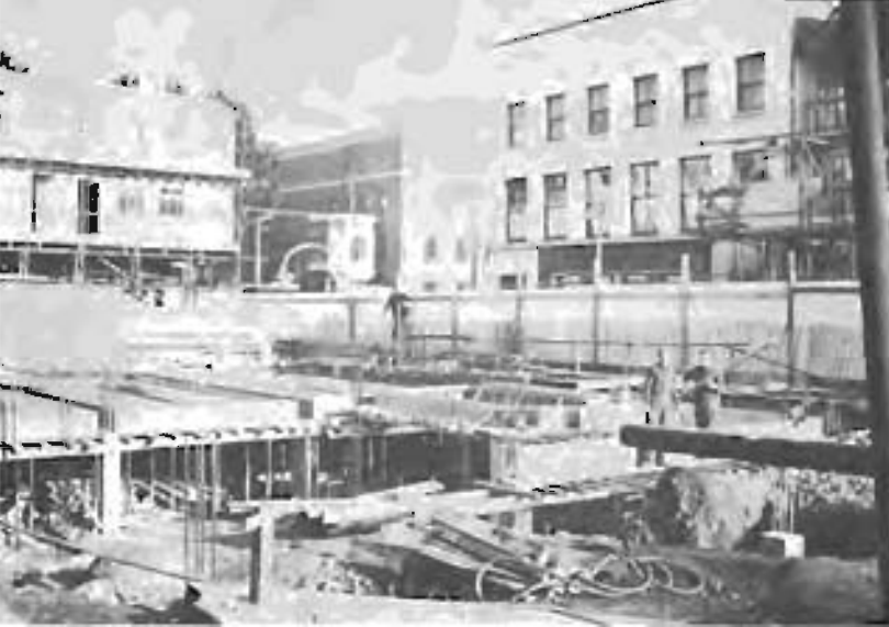
Work in progress on the new building
