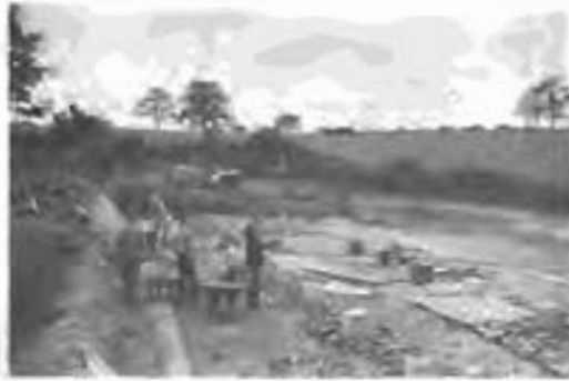
Work in progress on the extension of farm buildings
